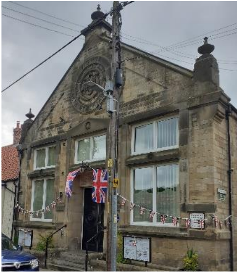
Scarth Hall, Staindrop Asset type: Building
